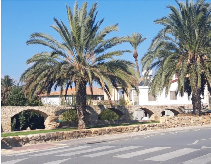
Fig. 50. Part of the Silahtar Aqueduct in Nicosia within the walls, near Famagusta Gate and very close to the Archbishop's Palace, 2020. © Evanthia (Evi) Tselika
