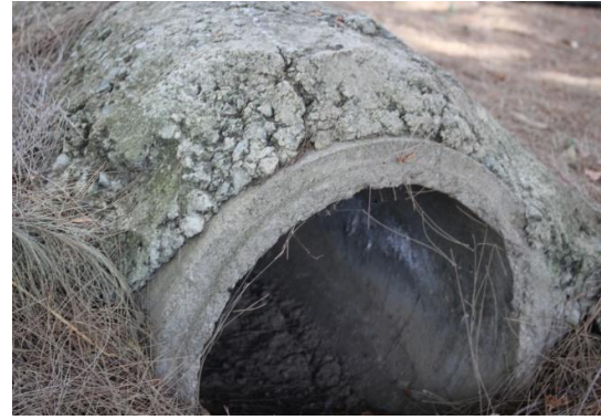
Fig. 19. Water tunnel in the Linear Park, Strovolos, 2020. © Evanthia (Evi) Tselika
