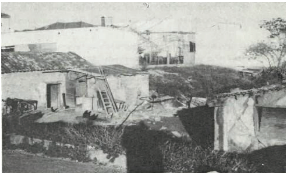
Traces of the medieval moat of Nicosia near Lykavittos Police Station.
